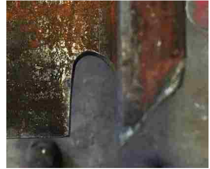
Figure 3.25: Completed weld access hole.
