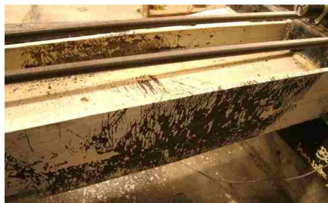
Figure 4.49: S col. severe yielding at 2.8% drift (Y3-OF/IF).
