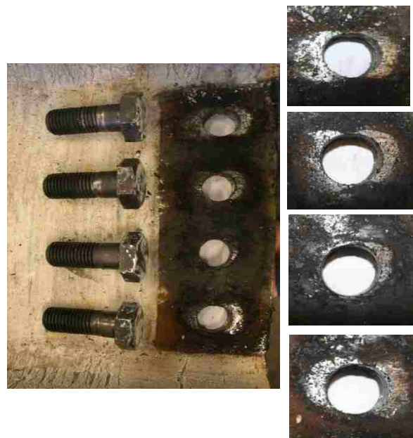
Figure 4.29: N beam web bolt hole elongation.
