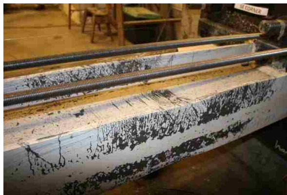
Figure 4.77: S col. severe yielding at 2.8% drift (Y3-PH).
