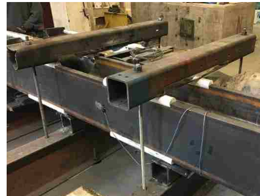
Figure 3.16: Installed out-of-plane restraints.
