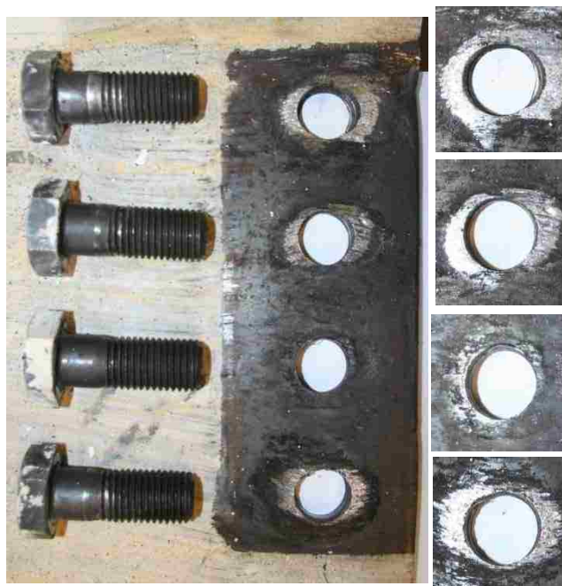
Figure 4.91: N beam web bolt hole elongation.
