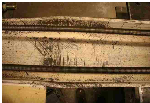
Figure 4.79: S col. moderate local buckling 3.0% drift (LB2-OF/IF).
