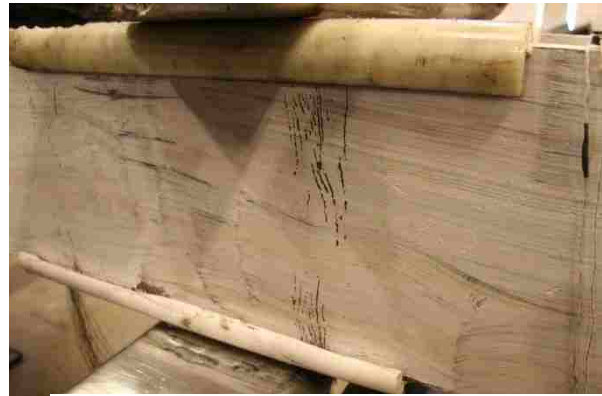
Figure 4.38: Beam OF initial yielding at 1.4\% drift (Y1-OF).
