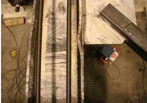
Figure 4.26: N column moderate local buckling at -3.3% drift (LB2-IF).
