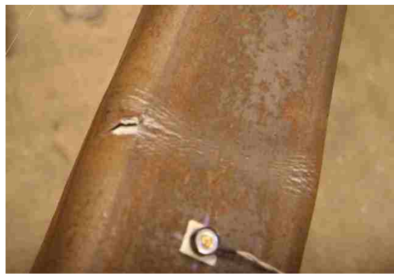
Figure 4.81: N brace crack/striations at -3.3% drift.
