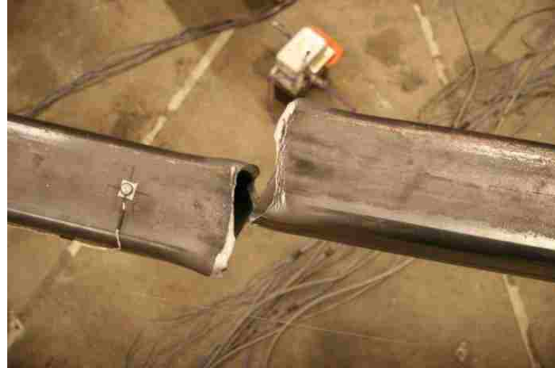
Figure 4.27: N brace fracture on second cycle at -3.3% drift (B4-BF).
