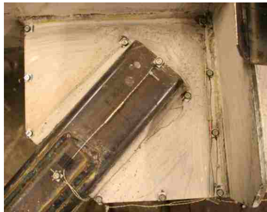
Figure 3.30: Optotrak LEDs on midspan gusset.
